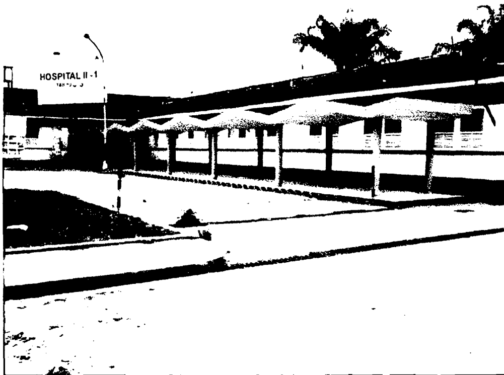
INGRESO PRINCIPAL AL HOSPITAL II
